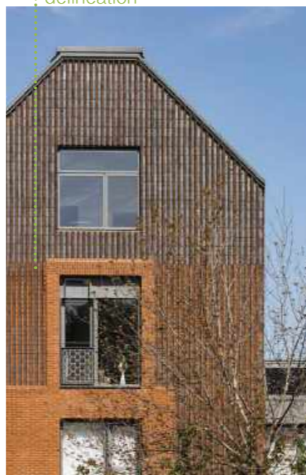
Brick variation and horizontal delineation
