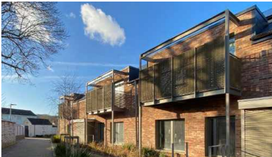
Challender Court - Passivhaus flats for Bristol City Council
