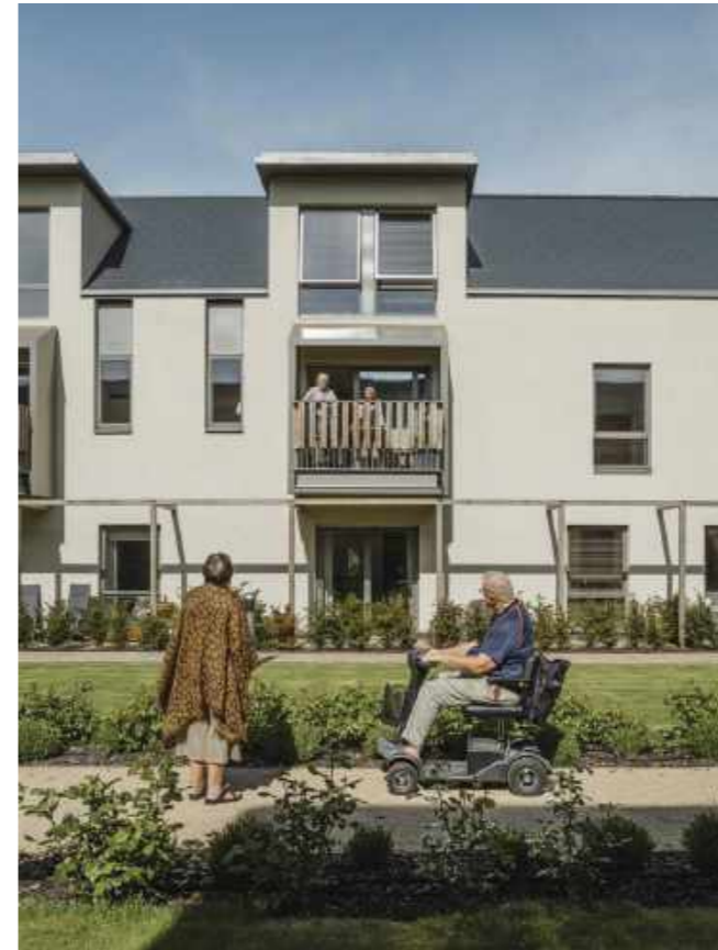
Render dormers creating usable 2nd floor areas whilst keeping eaves low
