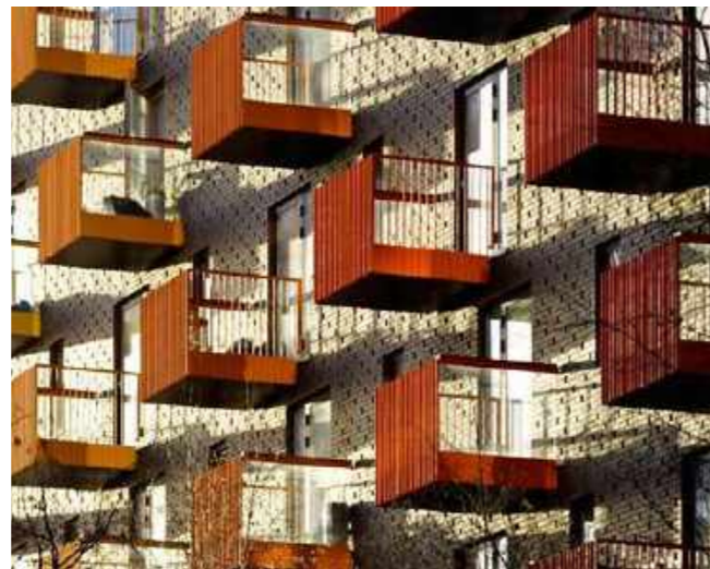
Coloured guarding to balconies
