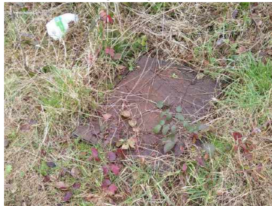
9. Existing services crossing the site
