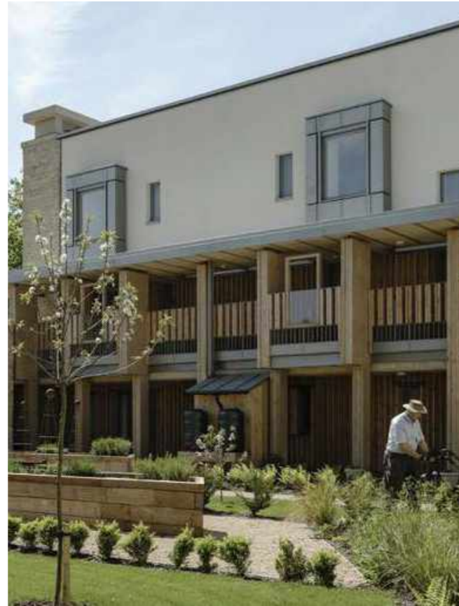
Timber structure for balconies and solar shading. Horizontal divides to break up vertical massing
