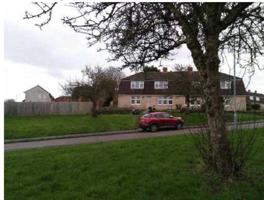
3. Adjacent property on Turner Gardens
