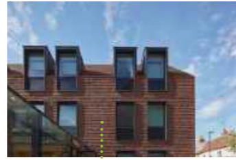
Hung tile roof and bays
